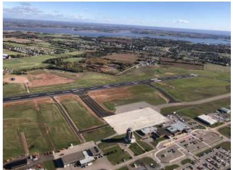
Charlottetown Airport Runway Rehabilitation Project
